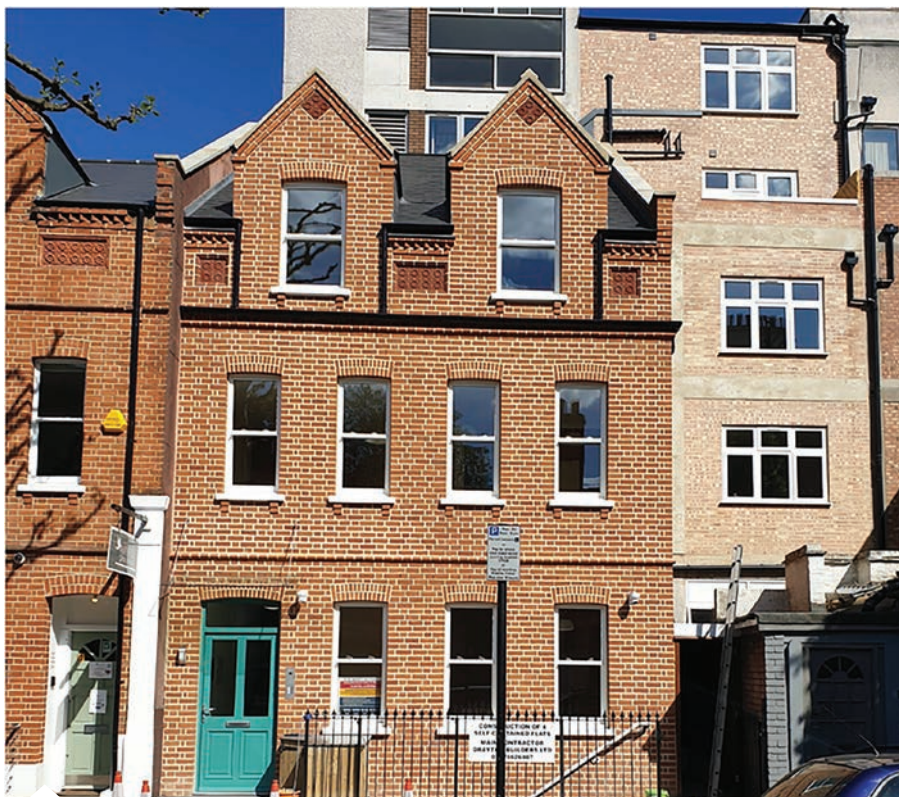
3 Ravenscourt Avenue - front budynku
